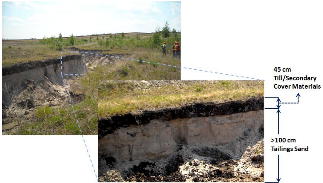
Figure 3.2. Soil cover system of the SWSS site.
