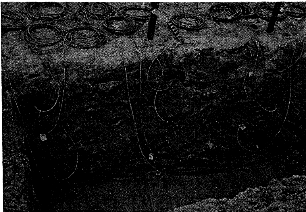
Figure 4.6 Photograph of Beta-97 sensors installed in brown till.
