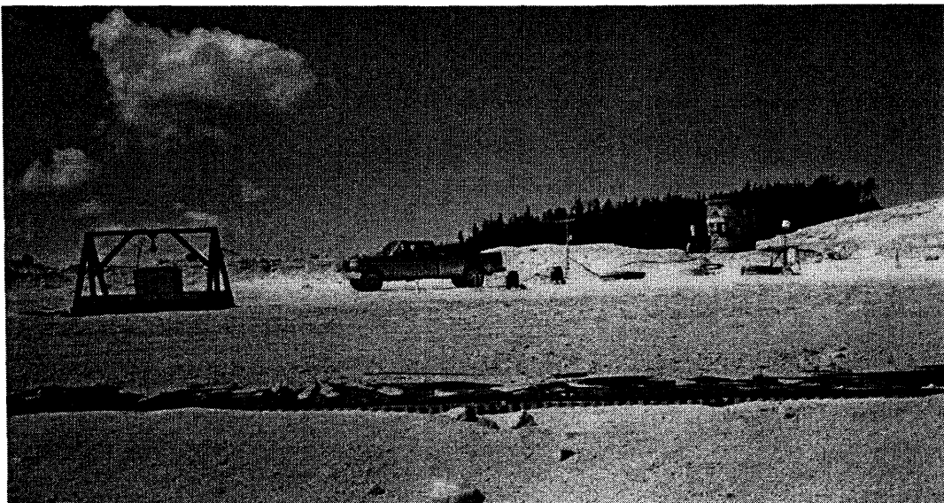
Figure 3.4 Photograph of the surface runoff collection culvert at HLTF. Looking north.
