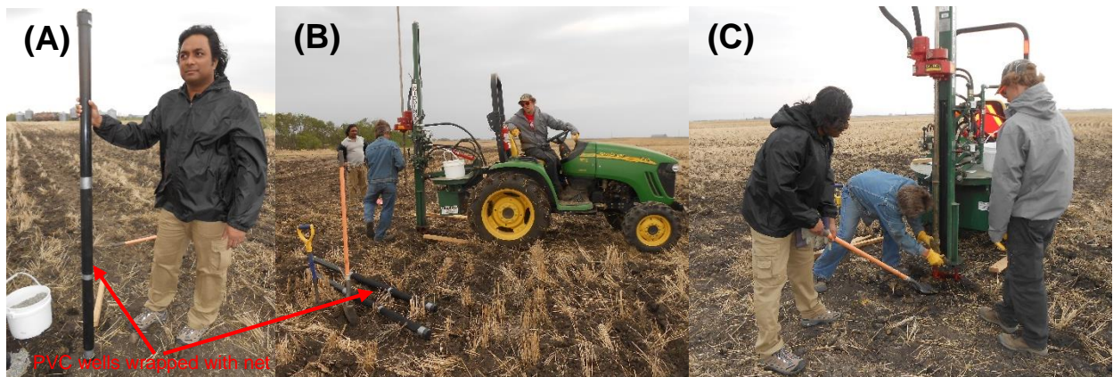
Installation of groundwater monitoring wells
