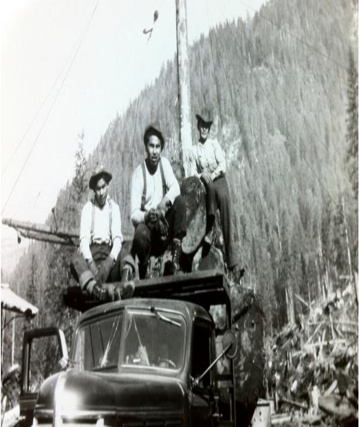
18 Tla'amin Logging Crew on logging truck- note the spar tree in the background (Courtesy of Tla'amin Treaty Society)
