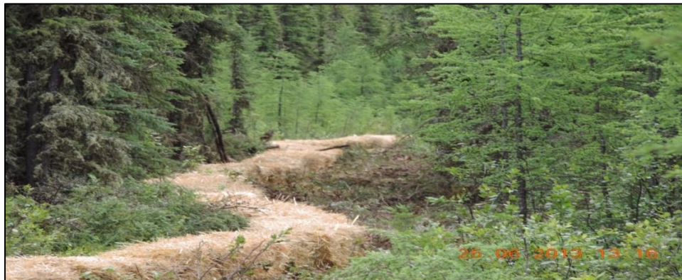
Figure C4 Hay bales were set around the perimeter of the spill site in order to keep the spill from spreading to the surrounding area (Gerbrandt 2013).
