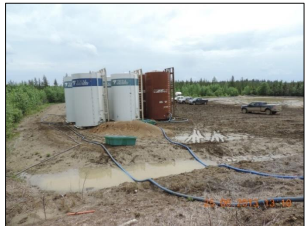
Figure C10 Once the produced water was cleaned, it was stored in these tanks until it could be safely pumped back into the spill area (Gerbrandt 2013).
