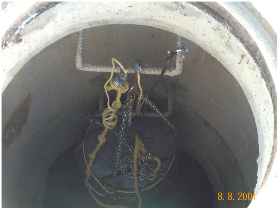
Figure 3.9 – Silverwood trunk water quality monitoring location – manhole with equipment installed.
