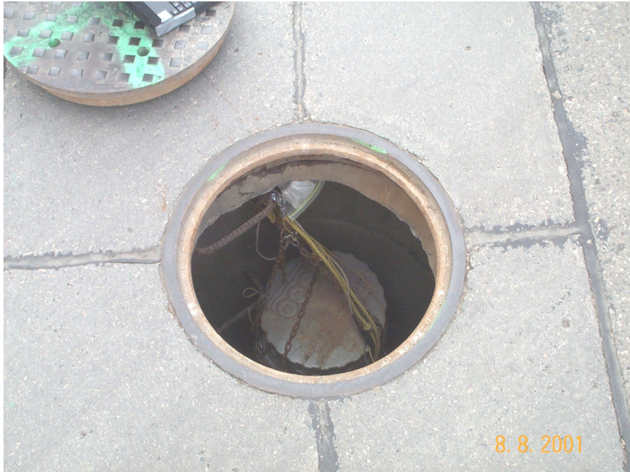
Figure 3.19 – Taylor Street manhole with sampling equipment installed.
