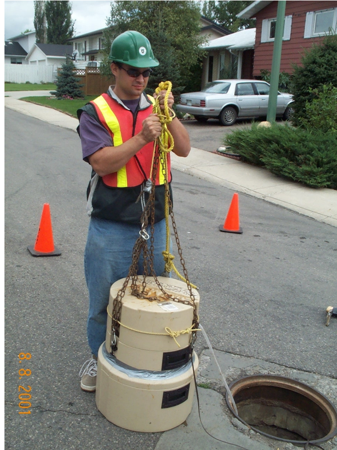
Figure 4.4 – Typical suspension harness setup.
