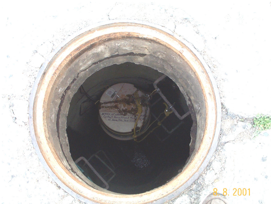
Figure 3.13 – Sturgeon Drive trunk 2001 water quality monitoring location manhole with equipment installed.
