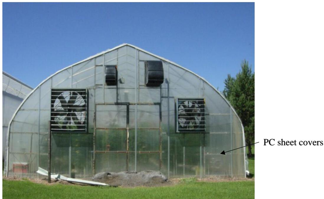
Figure 2.1 PC sheet covers used in traditional greenhouses
