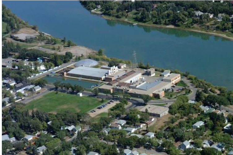
Figure 2.13 City water treatment plant picture
