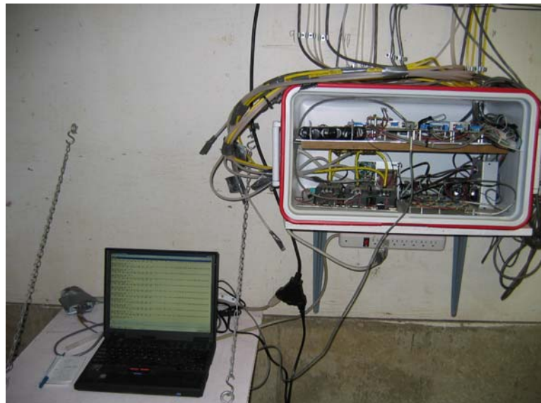
Figure A.2 The Measuring system installed in the swine barn.
