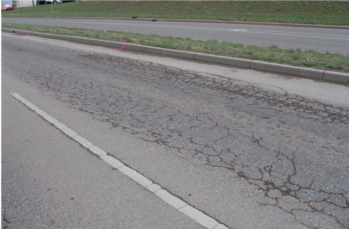
Figure 2.2 Structural Rutting (courtesy Dr. C. F. Berthelot)
