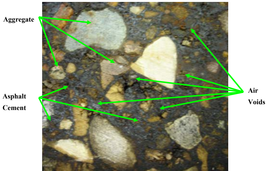
Figure 2.11 Saw-Cut Asphalt Concrete Surface
