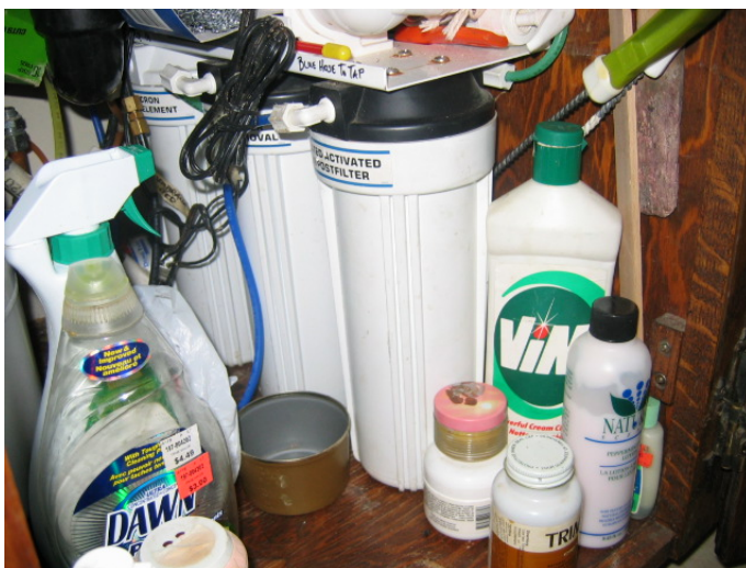
Figure 5.31 RO filtration system.
