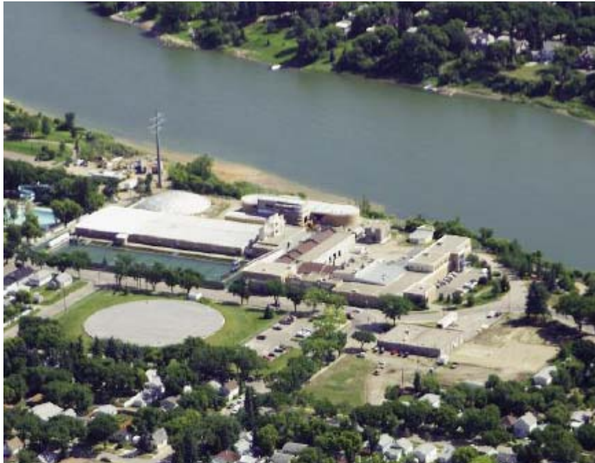
Figure 5.22 Aerial view of Saskatoon Water Treatment Plant (Keller 2006).
