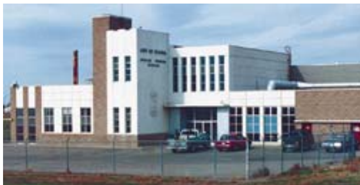
Figure 5.1 Buffalo Pound Water Treatment Plant.
