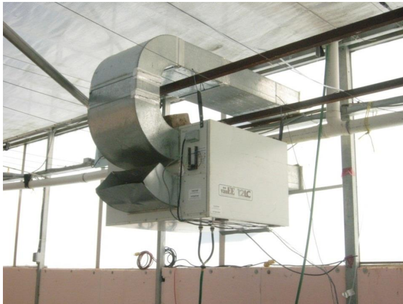
Figure 2.2. Heat exchanger installation.
