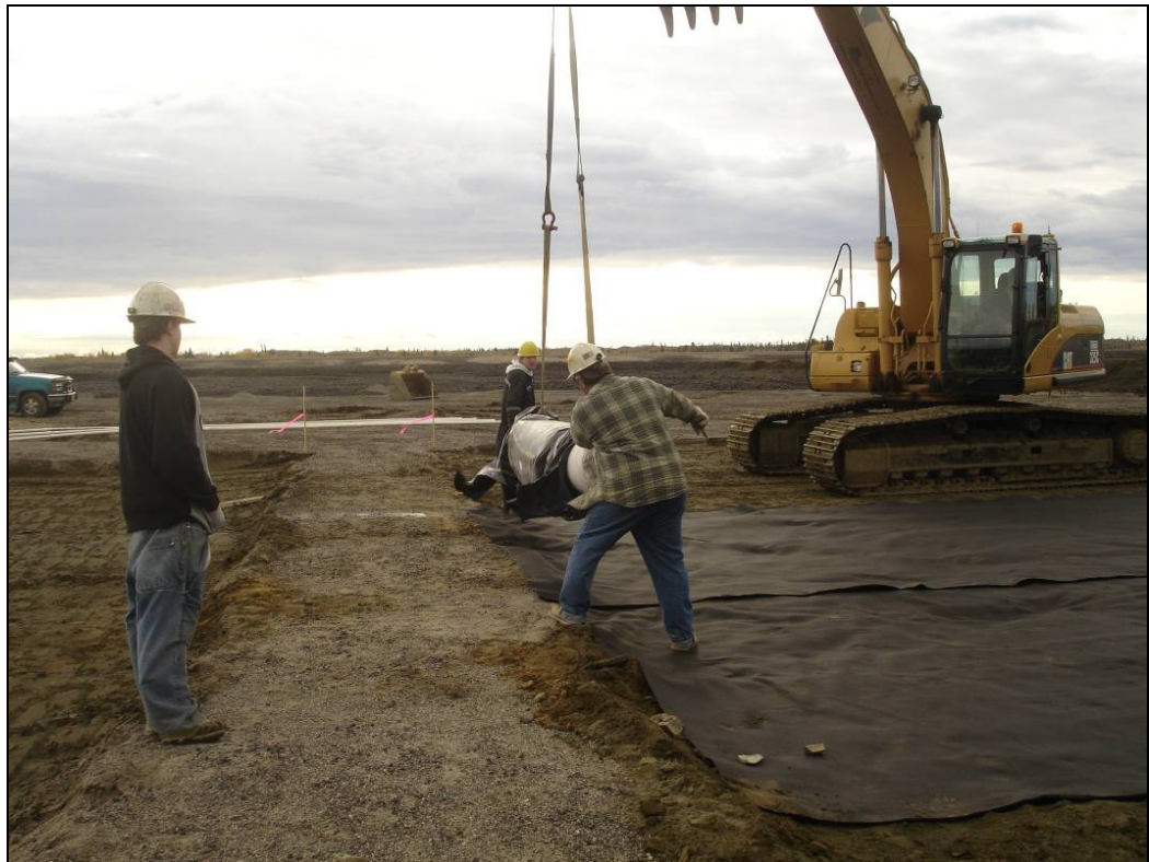
Figure 3-2 Placement of GCB over geotextile
