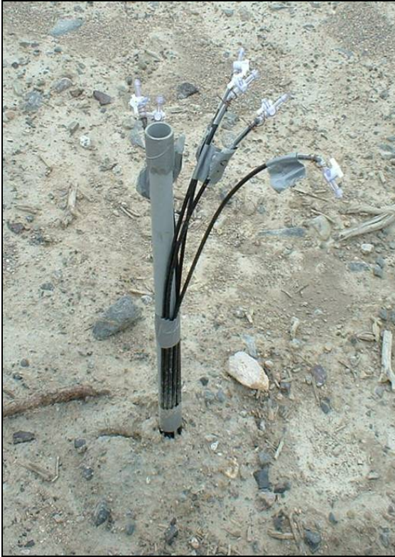
(a) Gas access ports after installation
