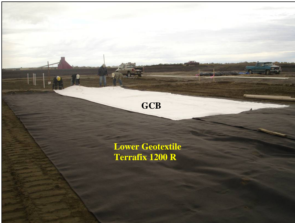
Figure 3-3 GCB placed on top of lower geotextile
