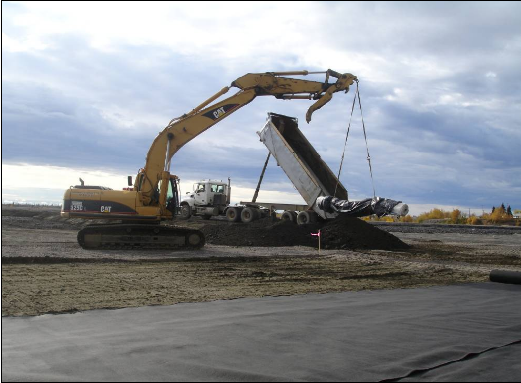
Figure 3-1 Transportation of GCB roll with excavator
