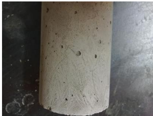
Figure 5.1 Close up view of a cylinder after de-molding, showing a crow-foot pattern indicative of early-age freezing
